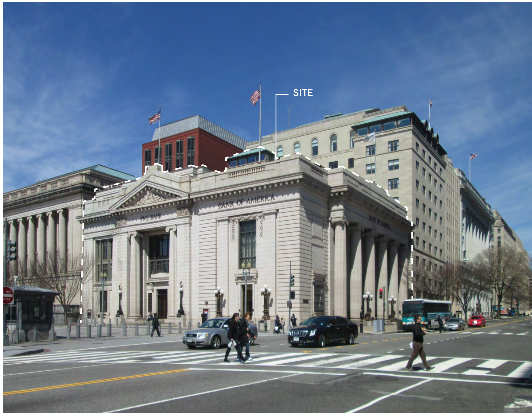
C. From Corner of Pennsylvania Ave. and New York Ave. Looking Northwest
