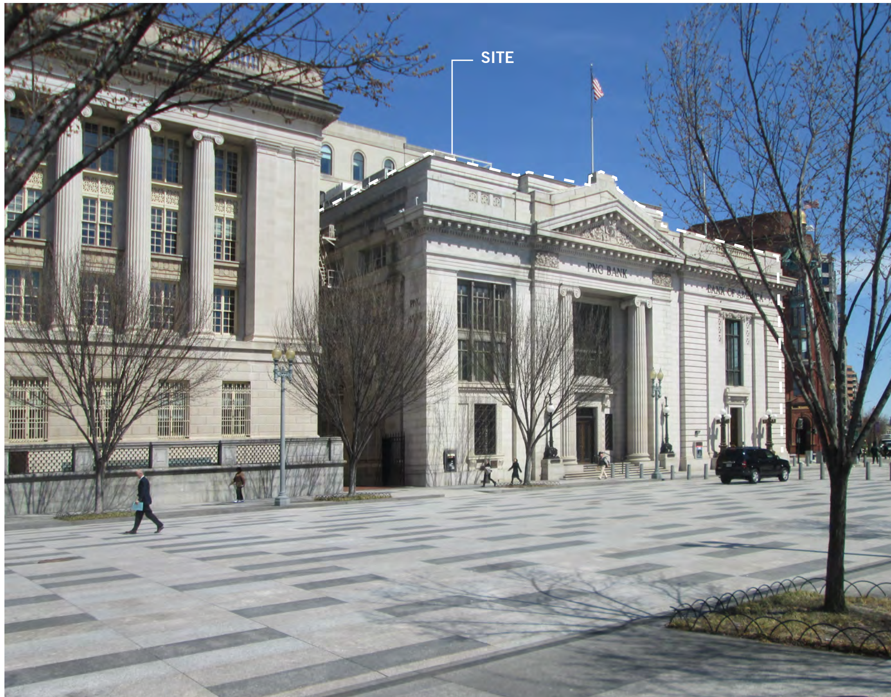
A. From Pennsylvania Ave Looking East
